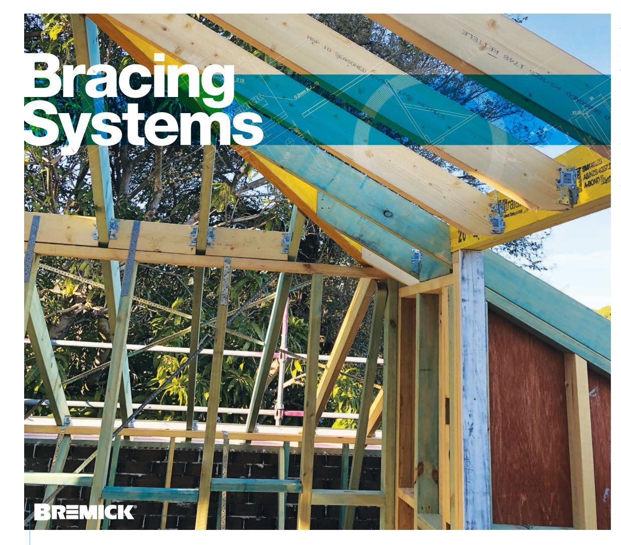
Bremick Bracing Systems (Strap Brace & Tensioners) are fully compliant to AS1684 and have been designed for structural bracing of residential timber and metal framed structures, while Bremick Hoop Iron is designed for use in general non-structural applications.
