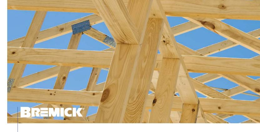
Bremick Nail Plates are ideal for joining timber in both structural and nonstructural applications. Tap-In Nail Plates, Mini Nails and Strap Nails are designed with pre-punched nails, while Nail-On Plates are designed with pre-punched fastening holes for use with nails or screws.
